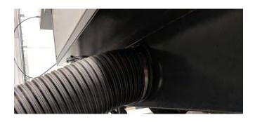
6" Exhaust tubing installed w/ hose clamp
